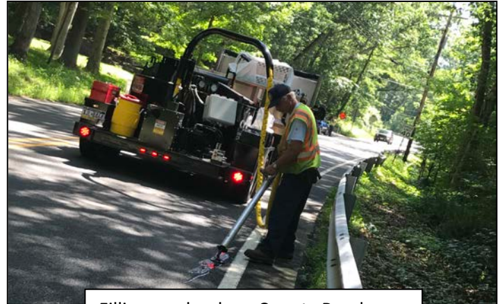
Filling cracks along County Roadways
